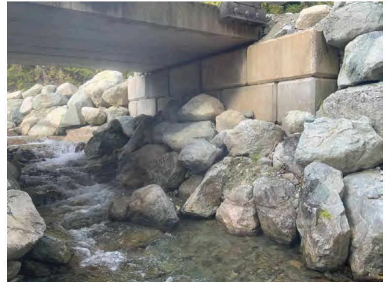
Left Bank Abutment when facing downstream
