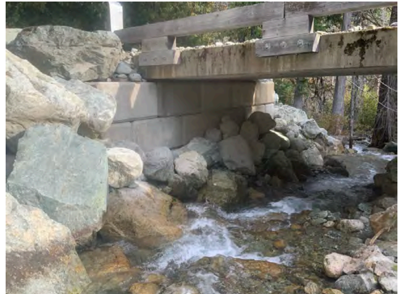
Left Bank Abutment when facing downstream
