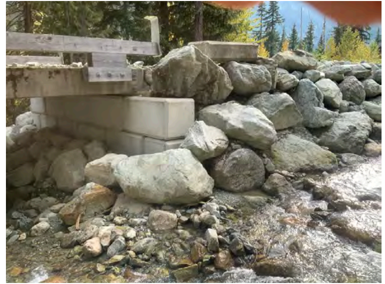
Right Bank Abutment when facing downstream
